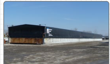
Second-stage curing enclosure allowing additional moist curing per MTO regulations.
