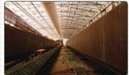
Protect forms & employees from the elements when preparing for the pour.
