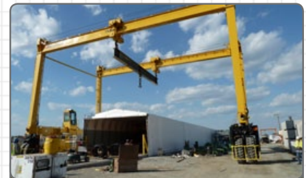
Full overhead & side access to girder forms.
